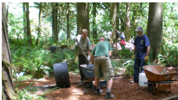
Service: Volunteers construct a new campsite
